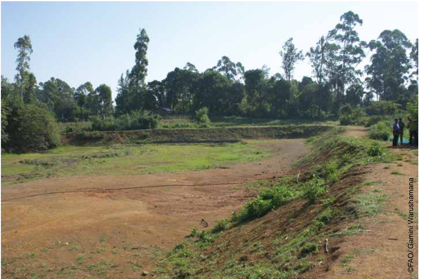
Renovated Kalubululanda Tank
